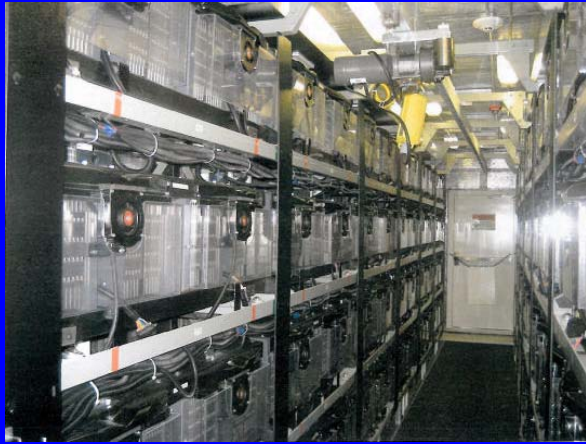
4 x 1MW / 15min Li-Ion in PJM. CA-ISO
