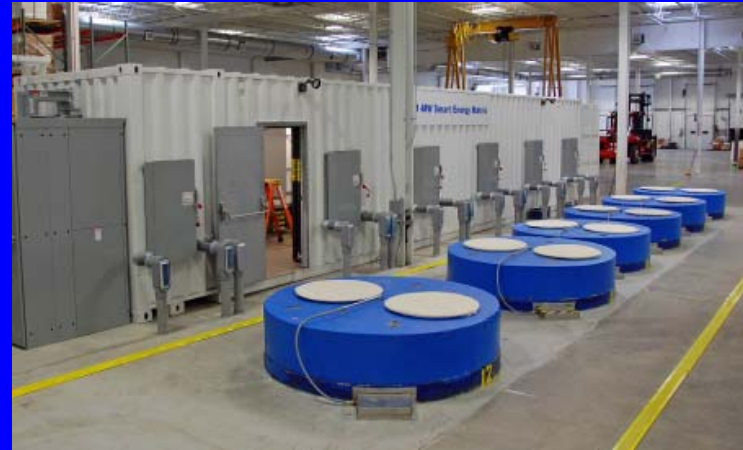
2 x 1MW / 15 min Flywheels in NE-ISO
