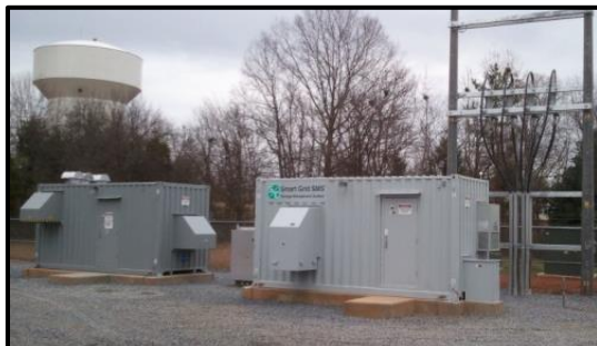
402 kW / 282 kWh Sodium Nickel Chloride Mt. Holly, NC
