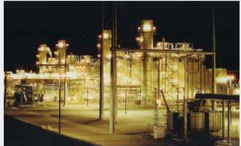
Union Power Station
